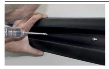
Drill and screw the base profile directly to the boat every 15/20 cm.
