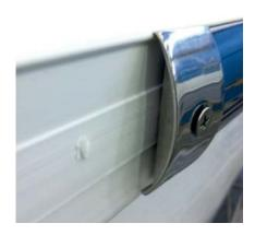
The drill spindle must not touch the countersink of the screw: we recommend inserting a plastic or aluminum stop buffer on the drill bit; this simple operation will prevent the iron material of the spindle from damaging the steel. It is advisable to apply silicone to the hole making screwing smoother and sealing the hole itself.
